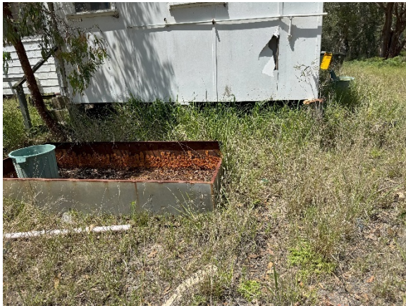
Photo 3: Small metal bund of former diesel tank.
